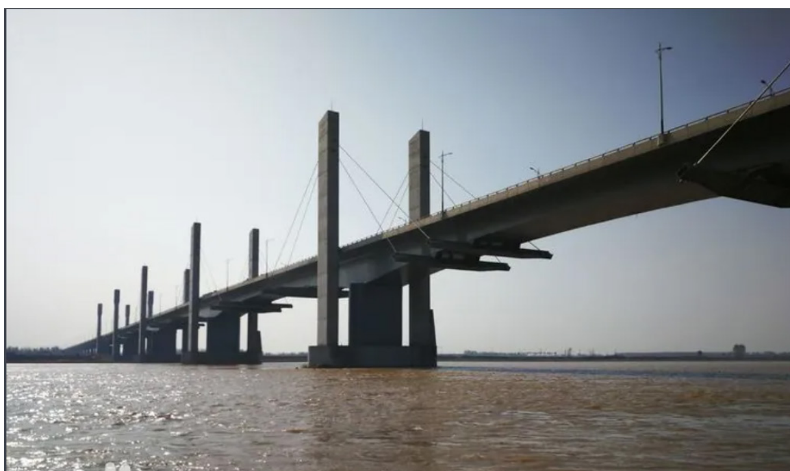
Fig. 3. Strengthened Dongming Huanghe River Highway bridge.
