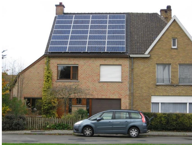
Fig.4.4.1 Photovoltaic panels mounted on the roof of a private household
