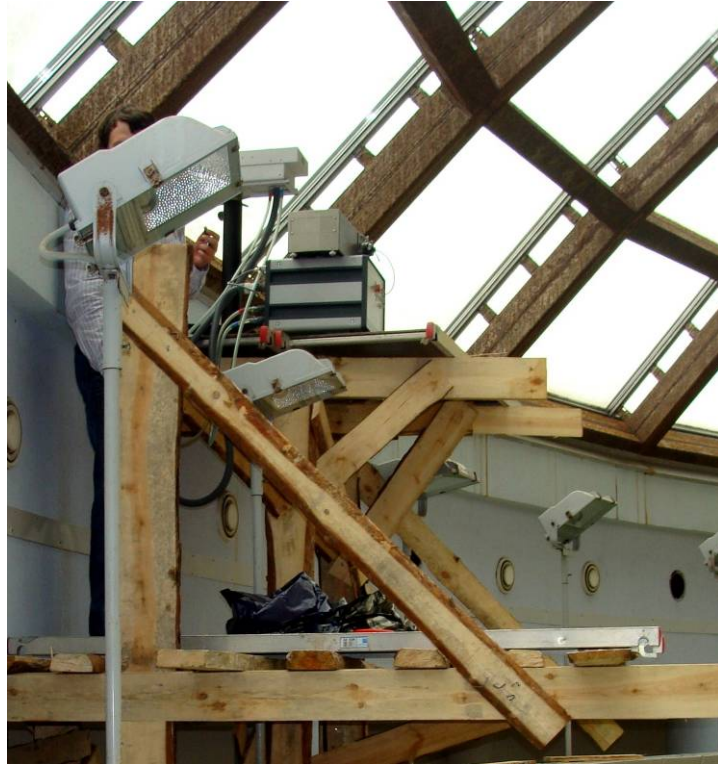
Fig 3. The examination of corrosionless metal in the aquapark.
